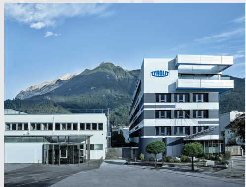
TYROLIT headquarters in Schwaz (Austria)
