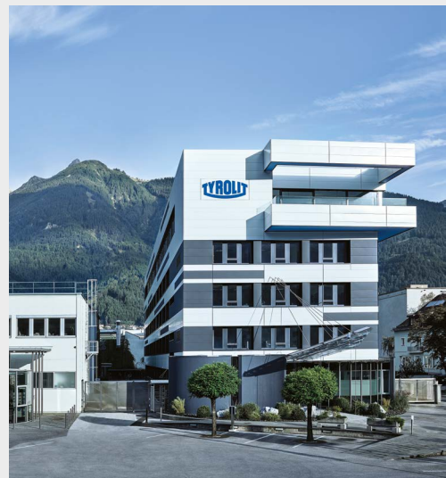
TYROLIT headquarters in Schwaz (Austria)
